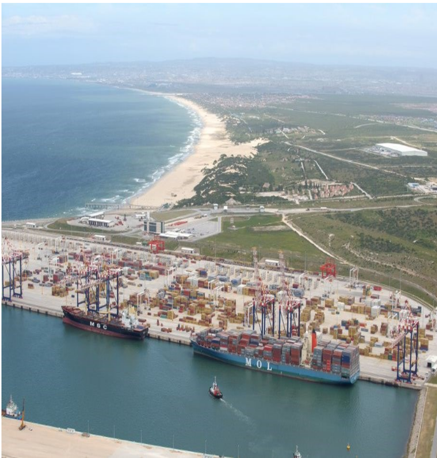
Picture: Port of Ngqura
